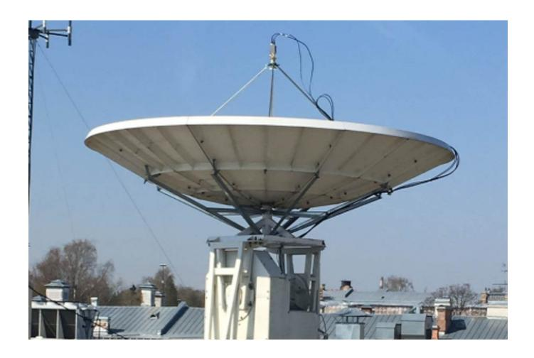
To date, the development of AIS has been completed and preparations for the assembly of two microsatellites have begun. The Radian 3.6 antenna-mast device for receiving AIS signals in the S, C and X frequency bands of the ground station for receiving and processing satellite information is located on the roof of the SPbPU NIC. The antenna device provides operation as a part of target radio lines of all available and prospective domestic microsatellite platforms.
